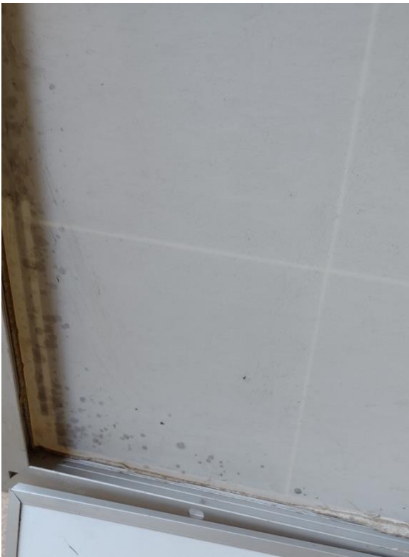
2110-CPV-001-017 *minor scuff marks in backsheet
